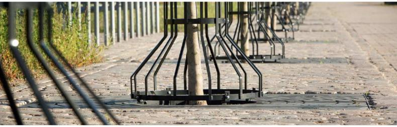
Redevelopment of the promenade on Kaistraße between the rail station and port. The modern RONDELLO® 2.0 tree grills are the perfect fit for the chosen cobbled surface and the surrounding contemporary architecture. The possibility of widening the opening inside the cast-iron tree grill from 700 mm to 1,100 mm in diameter over time and as the trunk grows ensures that the grill will remain in use for decades and that the tree pits and the soil around the trees will be protected against compaction.
