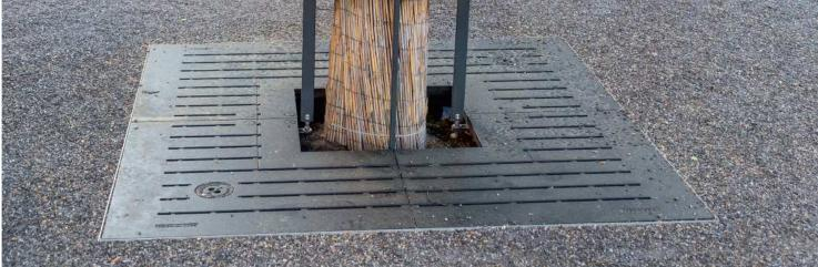
Renovation and upgrading of the pedestrianised zone on Postplatz in Zug. The LATERAL® 2.0 tree grills selected are ideal for both newly planted and existing trees since the inside opening can be adjusted as the trunk widens.
